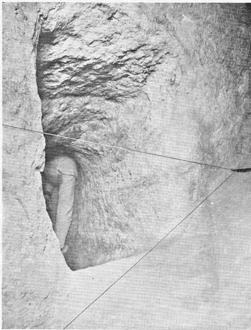
The lower end of the WELL-SHAFT of the Great Pyramid of Gizeh; showing the opening of the little passage which leads westward from the Descending Passage to the Shaft.
