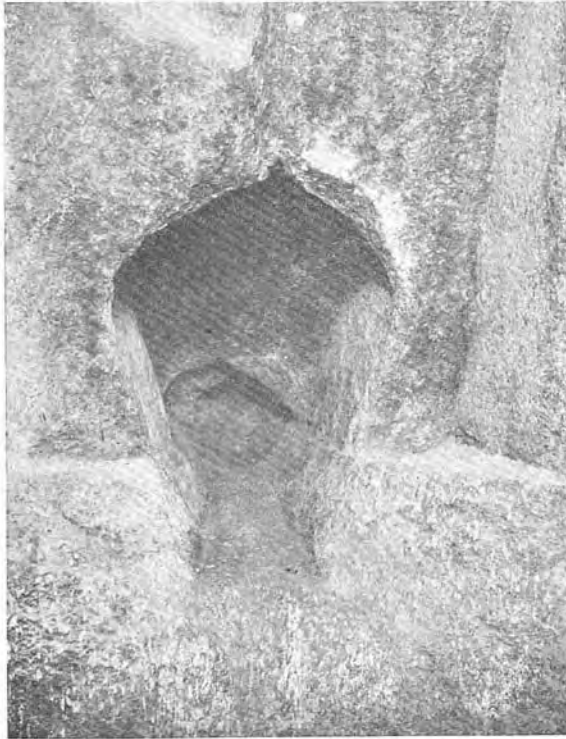
The mouth of the air-channel in the south wall of the King's Chamber.
