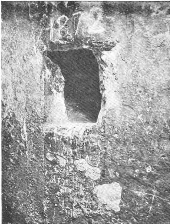
The north air-channel of the Queen's Chamber; showing part of the five-inch-thickness of once concealing stone.
