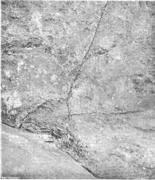
The bottom east corner at the lower end of the Descending Passage of the Great Pyramid of Gizeh, showing the hard natural concrete filling the corner.
