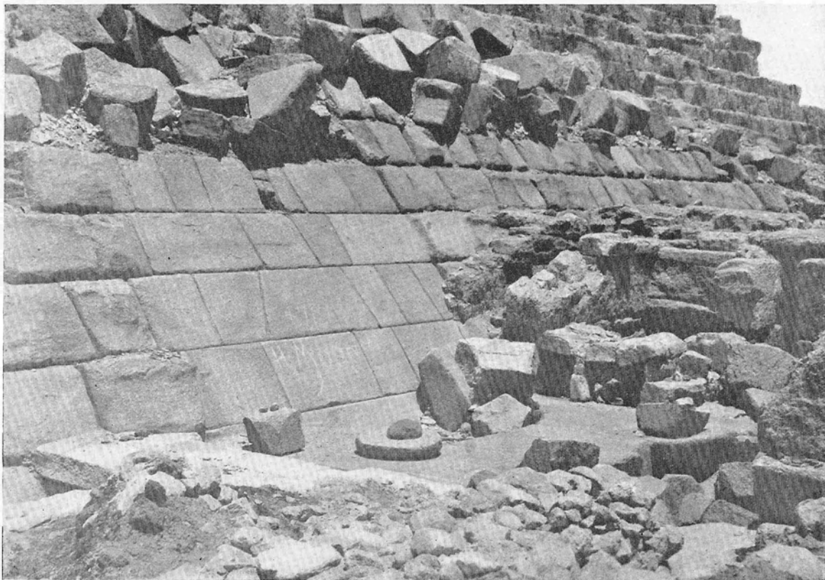
The east base of the THIRD PYRAMID of Gizeh; showing partly dressed granite casing-stones still in situ; also a portion of the granite pavement of the Pyramid's temple.
