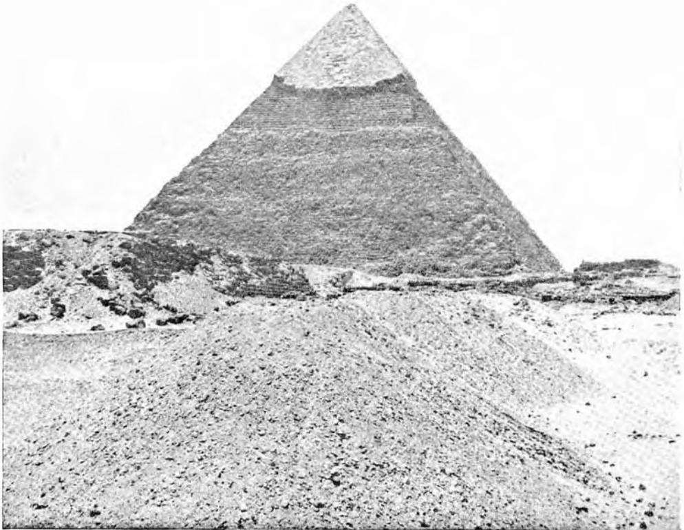
The north side of the SECOND PYRAMID of Gizeh; showing the remnant of the ancient smooth casing at the summit.
