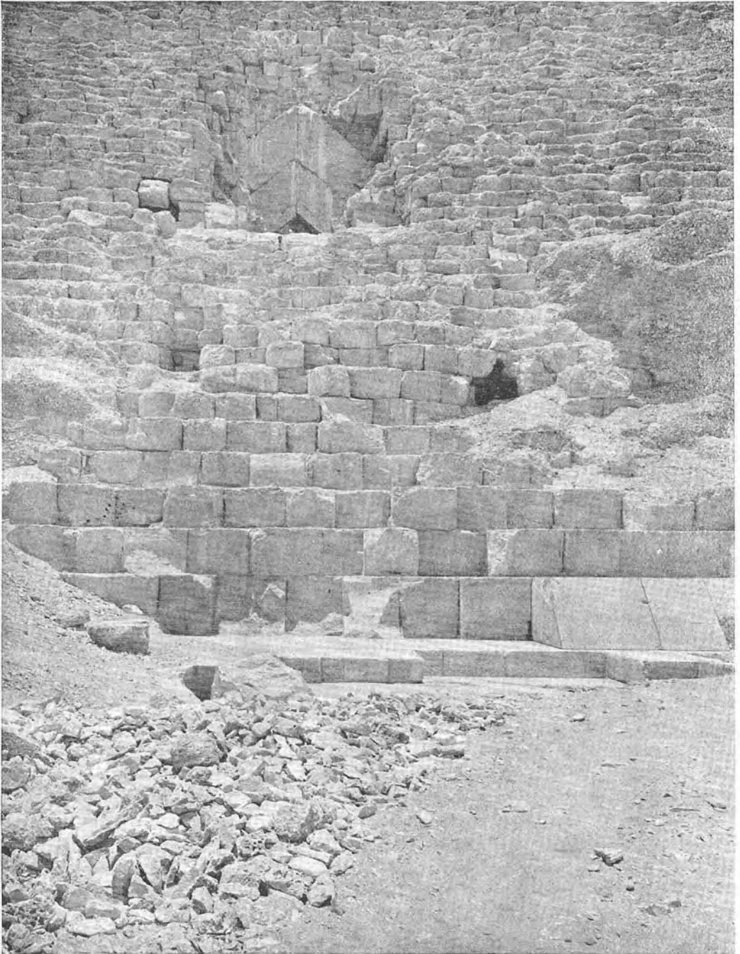
The MIDDLE of the NORTH BASE of the GREAT PYRAMID of Gizeh; showing the angle-stones above the Entrance, the casing-stones, and the entrance of Al Mamoun's forced passage.
