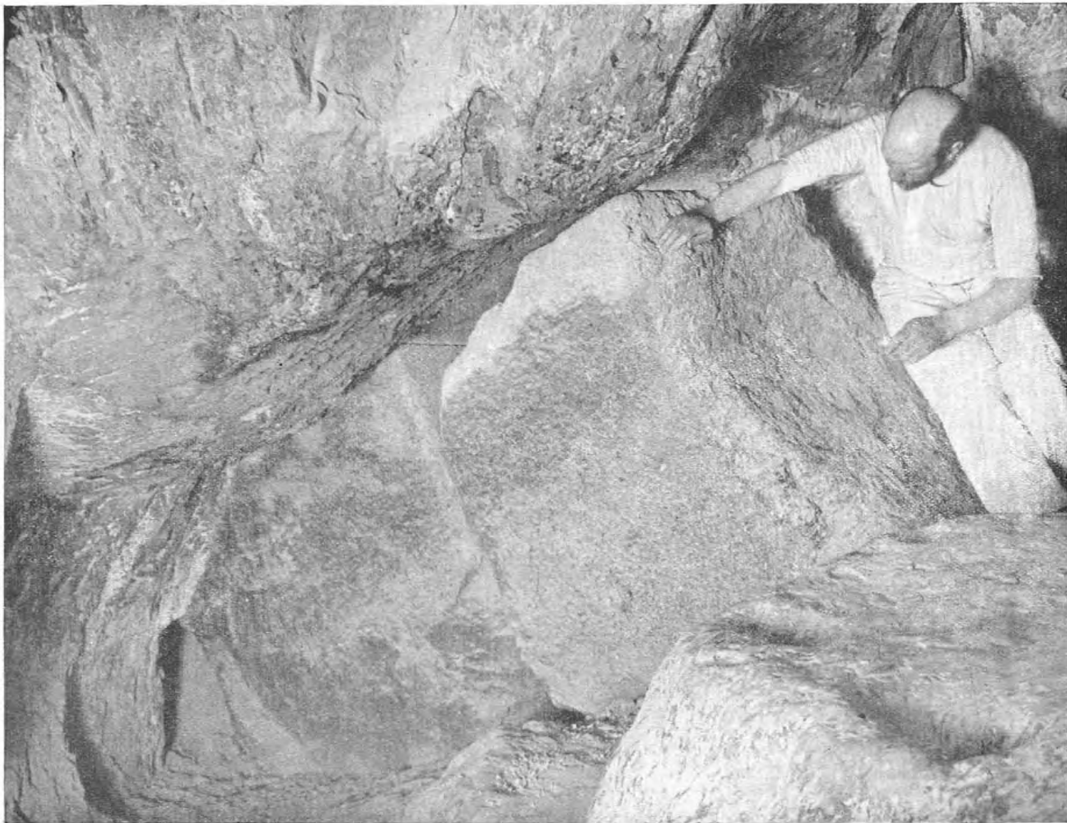
The upper south end, and portion of the west side, of the GRANITE PLUG which completely blocks the lower end of the First Ascending Passage in the Great Pyramid of Gizeh; showing two of the series of three great stones, hidden in the masonry for three thousand years, and exposed by Caliph Al Mamoun in the course of his excavations in the year 820 A.D.
