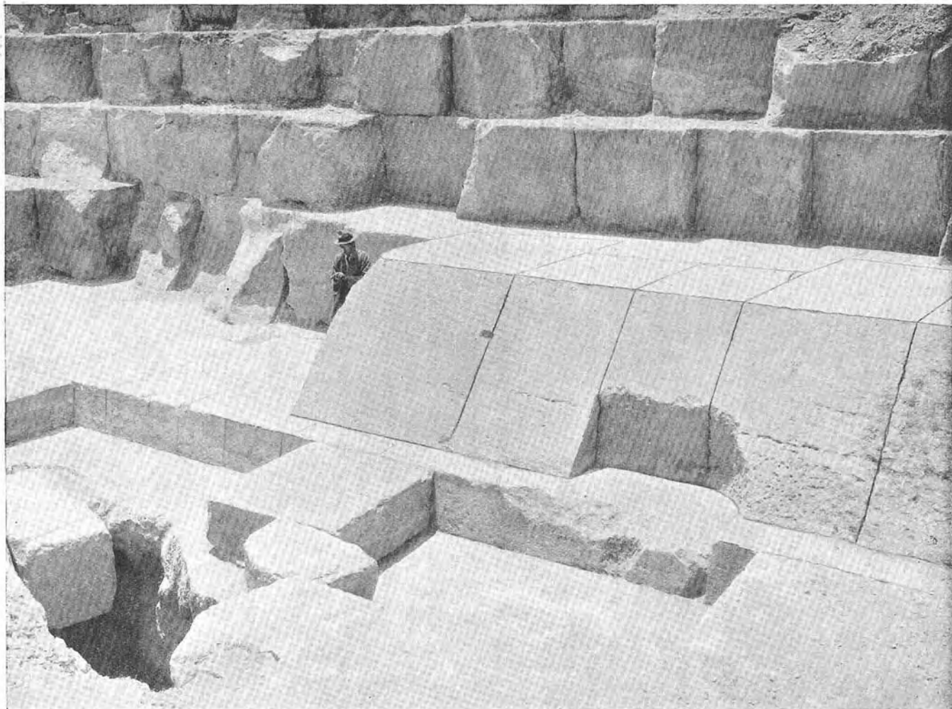
The best preserved of the CASING-STONES of the Great Pyramid of Gizeh; showing also the LARGE FISSURE in the rock, discovered by Col. Howard Vyse in 1837 A.D.
