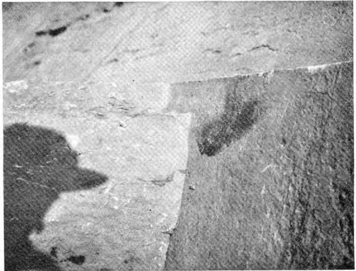
A fractured butt-joint between the pavement (on the left), and the bevelled front edge of the platform (on the right) in front of the casing-stones of the Great Pyramid of Gizeh.
