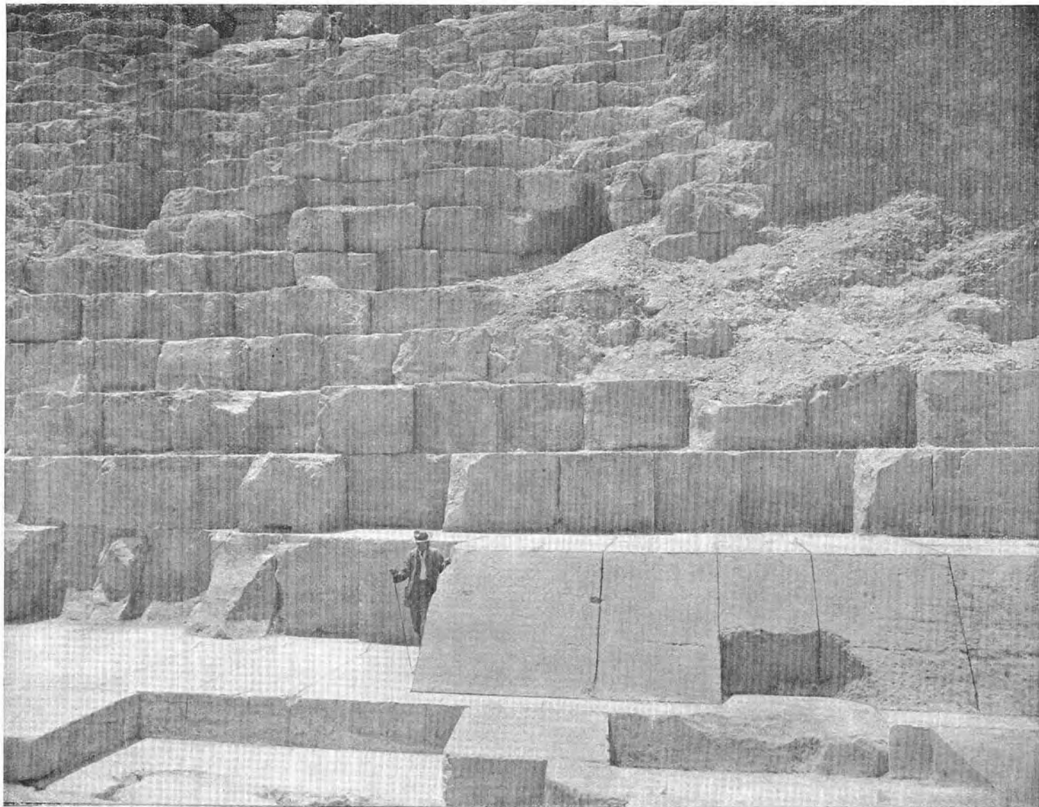
Mr. L. Dow Covington standing near his newly excavated CASING-STONES at the north base of the Great Pyramid of Gizeh.
