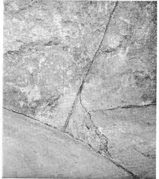
Same as Plate LI, but with the hard natural concrete removed from the corner.
