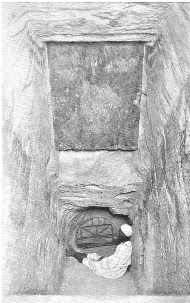
The IRON GRILL DOOR which closes the lower reach of the DESCENDING PASSAGE of the Great Pyramid of Gizeh; showing Judah sitting on the debris which concealed Petrie's granite block; also the lower butt-end of the Granite Plug which blocks the entrance of the First Ascending Passage.
