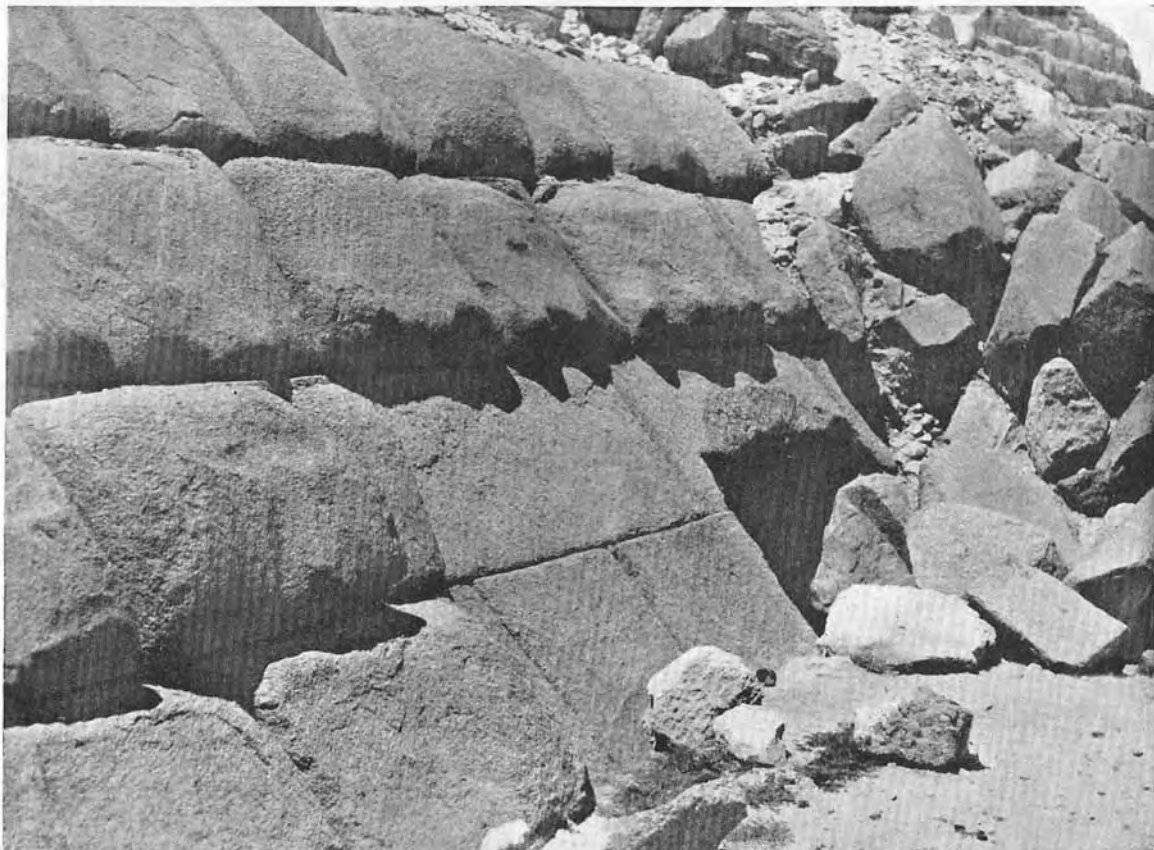
The ENTRANCE of the THIRD PYRAMID of Gizeh; showing a portion of the undressed granite casing-stones still in situ.
