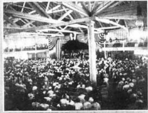
INTERIOR - CELERON AUDITORIUM
